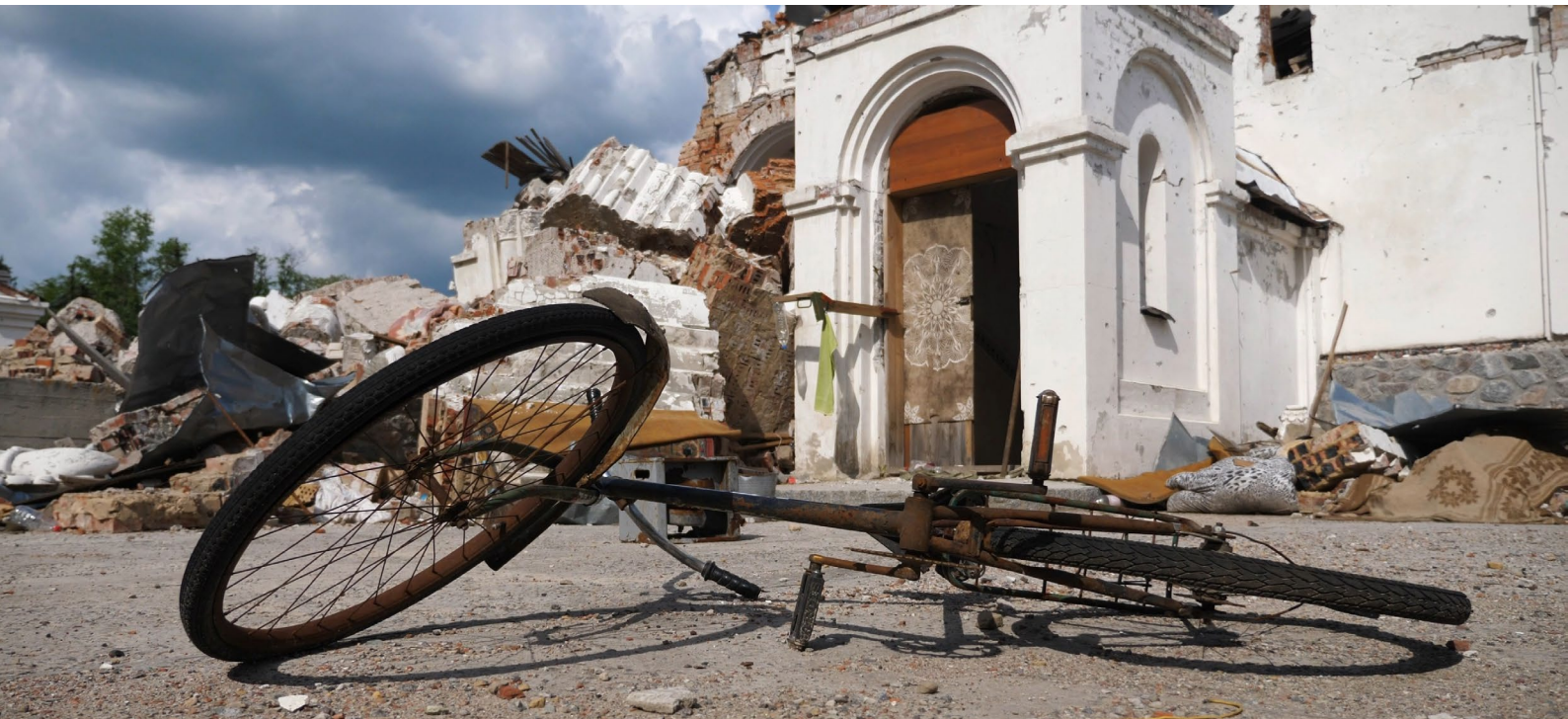
View to burned bike against the background of destroyed church at Kharkivska oblast. Ruined building after bomb attacks on ukrainian territory from russia army. russian invasion of Ukraine. Photo: Shutterstock.com
